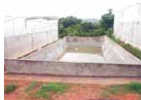
Lining of tank reinforced plastering on silpauline (top); finished lined tank (bottom left); check dam in Kaju Nallah watershed (bottom right)
