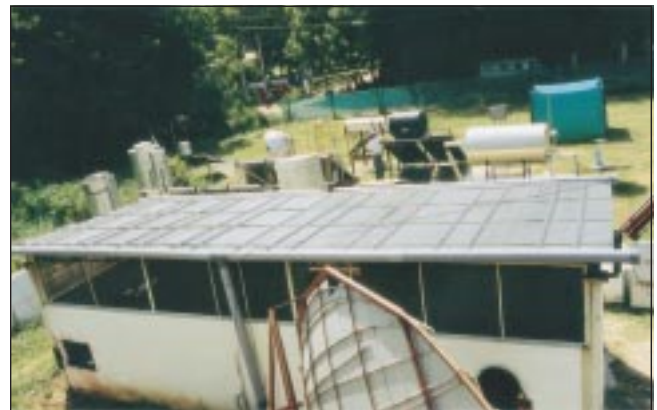
Roof integrated unglazed solar-air heater. This costs around Rs 1,000/m 2 . Its single module evaluation recorded a temperature rise of 15°C.
