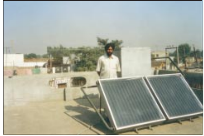
Flat-plate type solar-water heater. This heats 100 litres of water up to 55-60° on sunny days in winter at Ludhiana. Overnight drop in temperature of water was less than 5°C.
